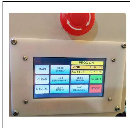
Figure 3 Typical settings for bringing cleaning fluid through the lines.
